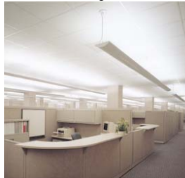
Photo: Courtesy of Litecontrol
