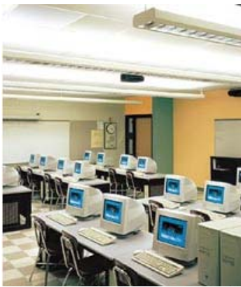
Suspended luminaires in this classroom illuminate the ceiling but also provide lighting to the work plane.
